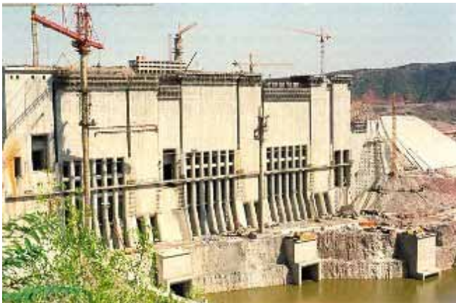
Tailrace tunnel discharge portals (to a common plunge pool)
