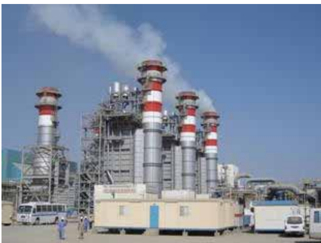
Sohar Combined Cycle Generation Units as seen from Desalination Plant
