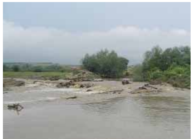
River flowing across road embankment after bursting its banks
