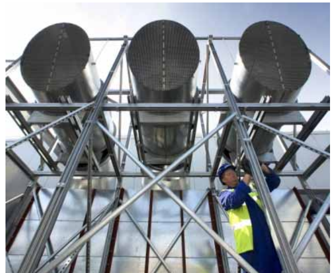
Preparing for cladding to HVAC exhausts, HQ Building, Sakhalin
