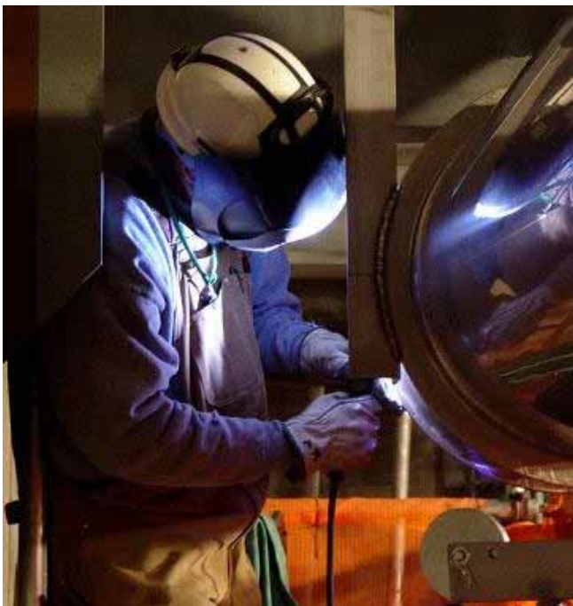
Welder working on a HVAC system, HQ Building, Sakhalin Island, Russia
