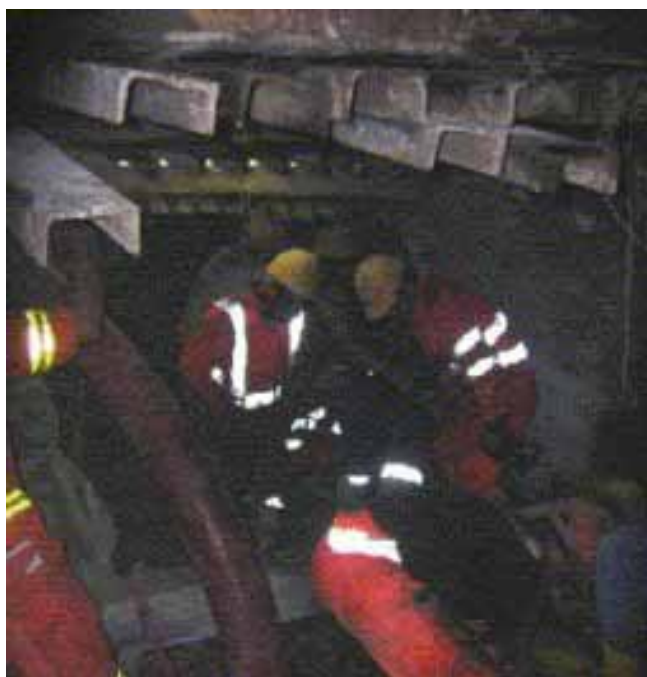
View of Pre-support Heading to Tunnel (ICC, 2004)
