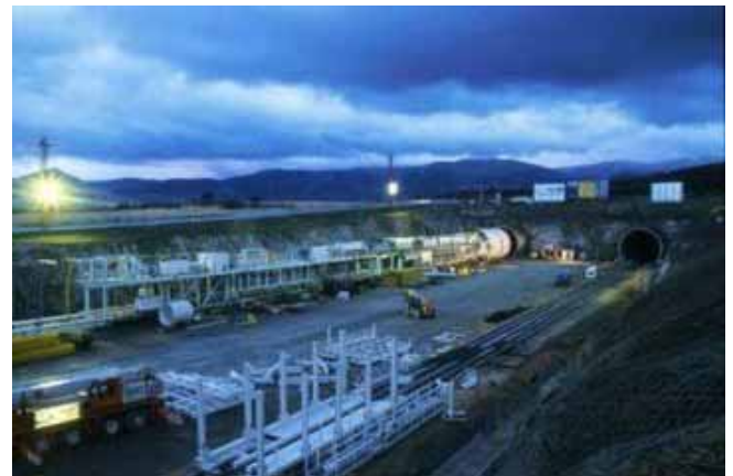
Erection of TBMs at Tunnel Portal
