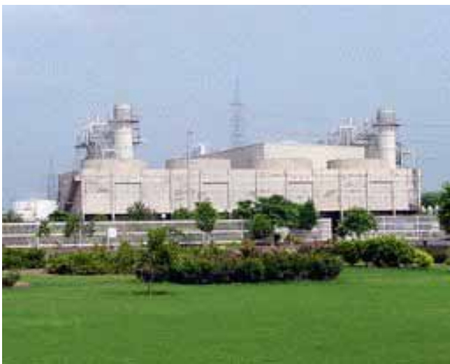
Fauji Kabirwala 155MW Combined Cycle Power Station, Multan, Pakistan.
