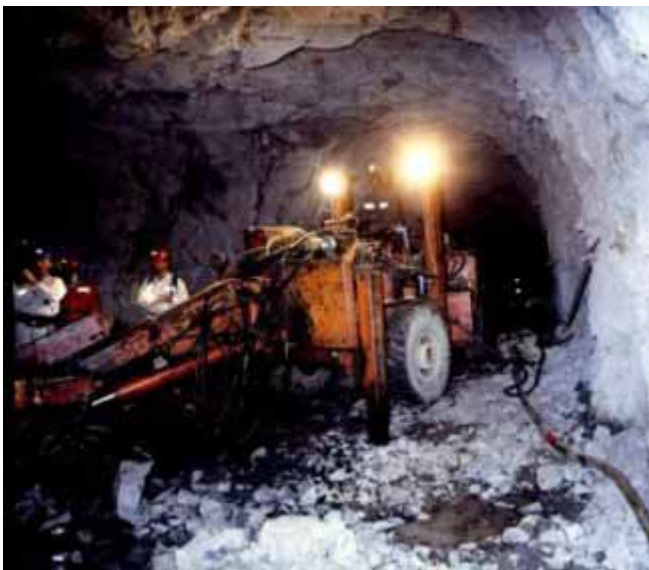
Drilling blast holes for next advance (round).
