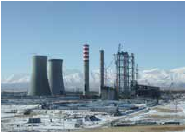
Power station under construction.
