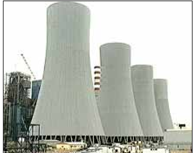
Cooling Towers to the Afsin Elbistan “B” Power Station (under construction).
